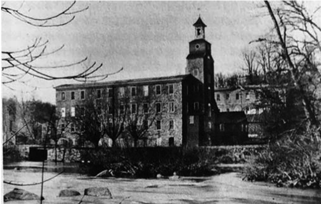
Figure 1. Photograph of Old Woolen Mill (1812) on the grounds of the duPont Powder Works. It represents the general typology of mill buildings with its masonry facade, narrowness, and numbers of windows. The building now accommodates the Hagley Museum in Greenville, Delaware. Courtesy of the Hagley Museum and Library. 6
